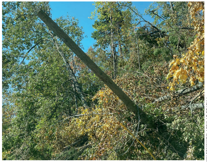
In the Rocky Bottom area, every power pole was broken or leaning due to torrential rain and high winds.
