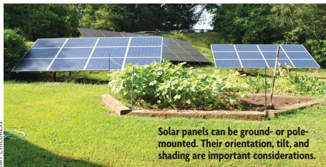
Solar panels can be ground- or pole-mounted. Their orientation, tilt, and shading are important considerations.
